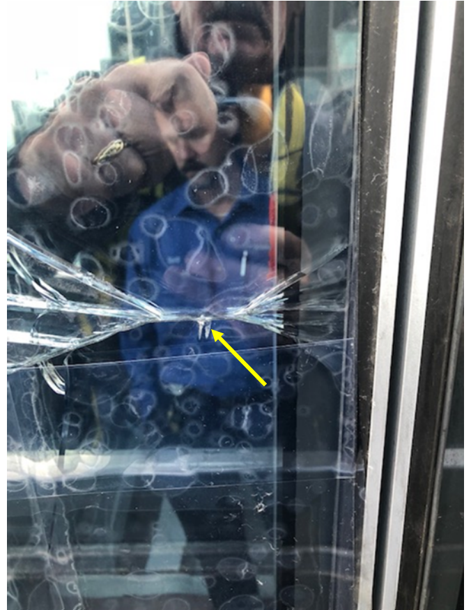
VIEW FROM EXTERIOR, AT SOURCE BREAK
