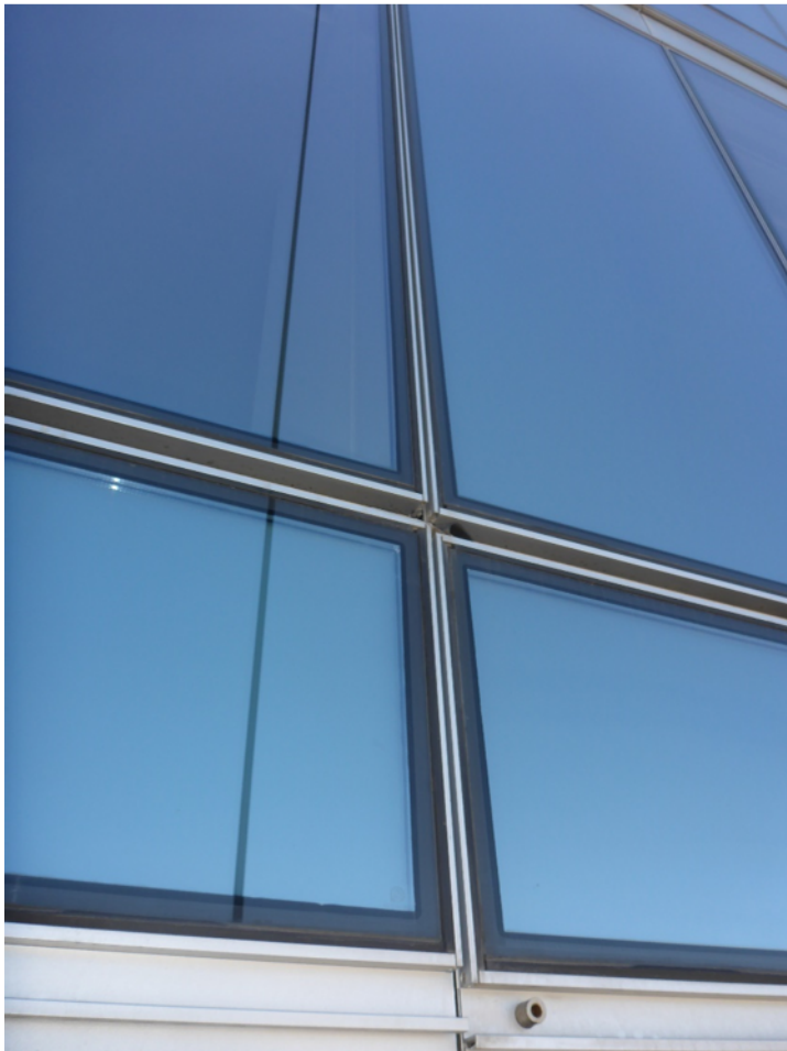
TYPICAL PANEL OFFSETS OBSERVED
