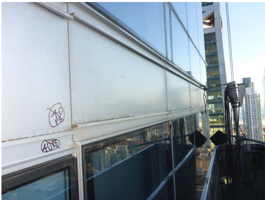
PRE-INVASIVE TESTING OBSERVATION OF SHIFTED PANELS
